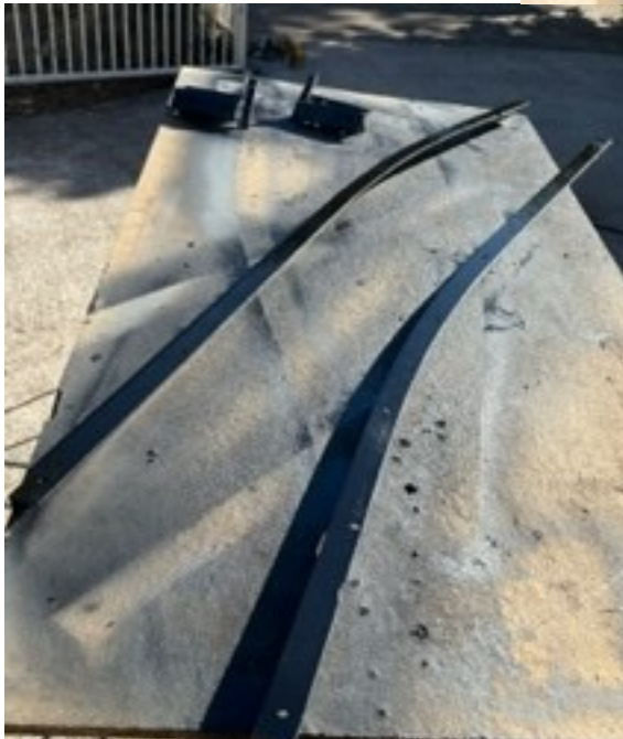
Above and adjacent: The angle iron sill edging and the front supports cleaned and new steel welded into them
