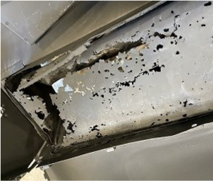
Above: Sandblasted battery box
