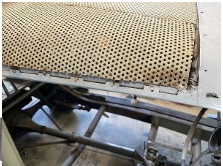
And on the roof
