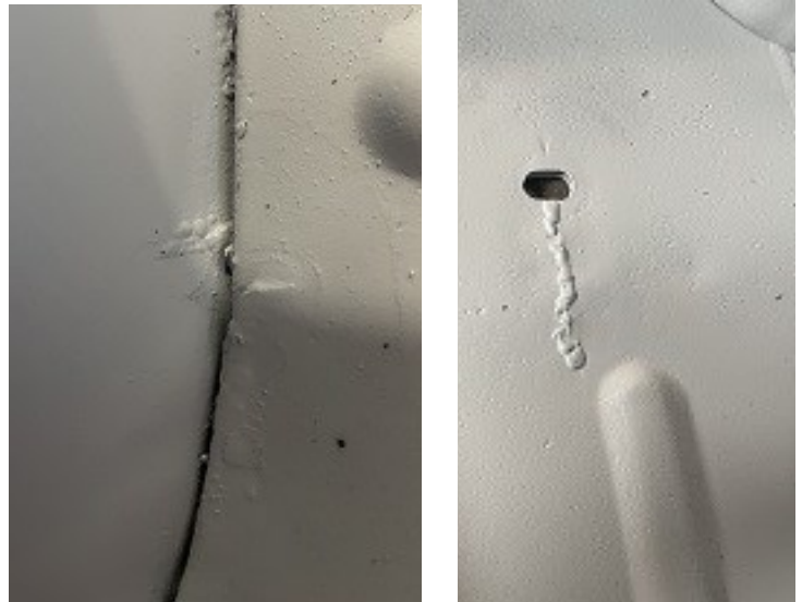
Above: Tub floor welded from underneath as well as above
